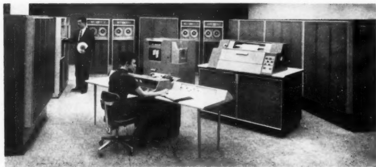
HONEYWELL 800 by Minneapolis-Honeywell Regulator Company is a transistorized model featuring an optimum word length, expandable magnetic-core memory (4,096 words to 32,768 words), high-speed magnetic tape units (peak transfer rate 96,000 decimal digits per second), and a wide range of both on-line and off-line input-output devices.
